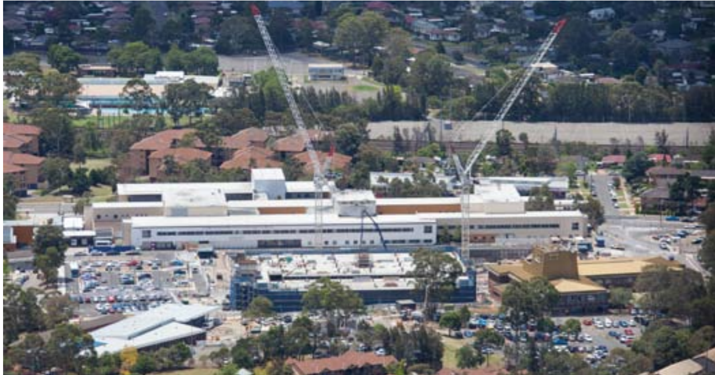
Blacktown Clinical Service Building Aerial
